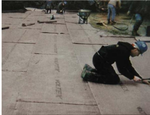
*Bentonite panel system: note nailing and poor seams*
