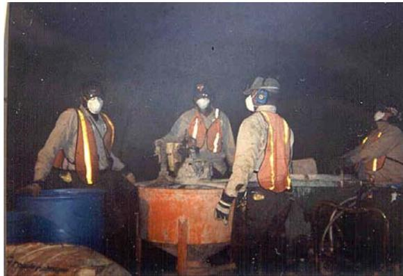
*Typical portable mixer and injection pump for particle grout*
