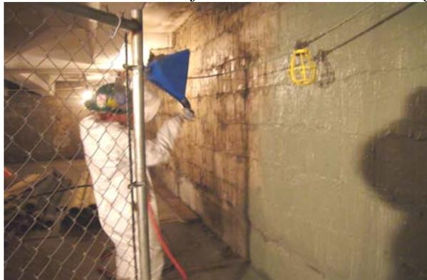
*Application of Masonry coating with hopper gun*
