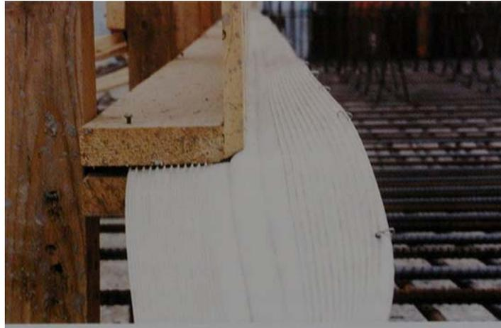
*Typical installation of vinyl or PVC waterstop: Note end is folded over*
