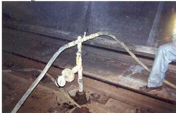
*Typical injection port for particle grout placement outside of the structure*
