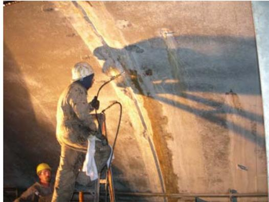
*Injection of chemical grout for sealing a construction joint*
