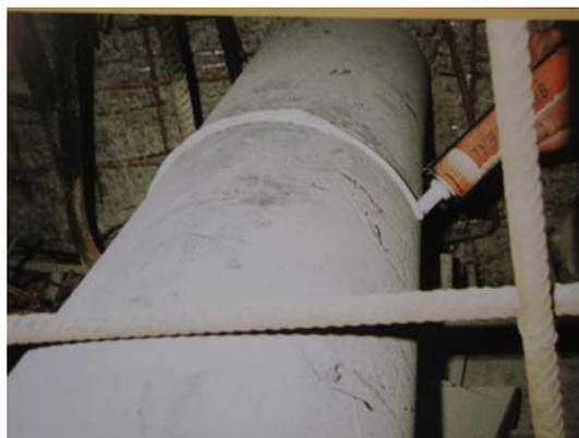
*Typical installation of gun grade swelling rubber on pipe penetration*
