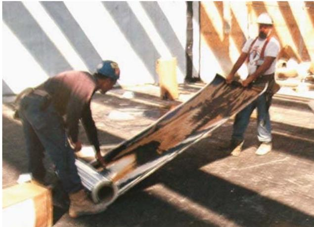
*Self adhered sheet membrane: note backing at edges of sheet*
