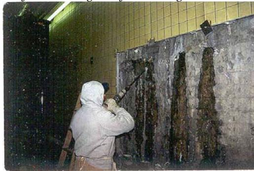
*Injecting a chemical grout in a horizontal joint note the grout return from joint*
