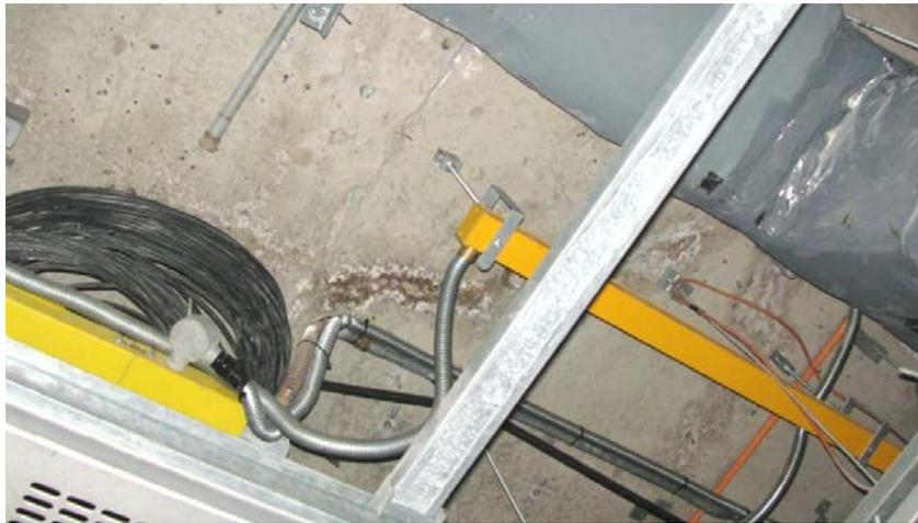
*Harbor Front MRT Station (Singapore): Note Leaking crack*
