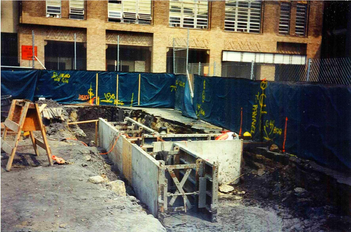
Photo 1: Formwork for guidewalls.
