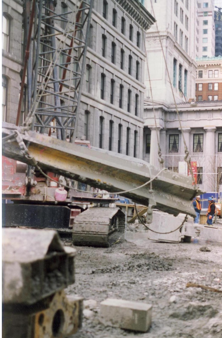
Photo 4: Typical chisel for rock and obstruction excavation (note 'V' nose end-stop, bottom left corner).
