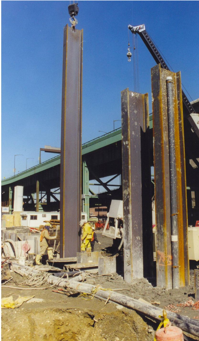
Photo 15: Setting soldier piles.
