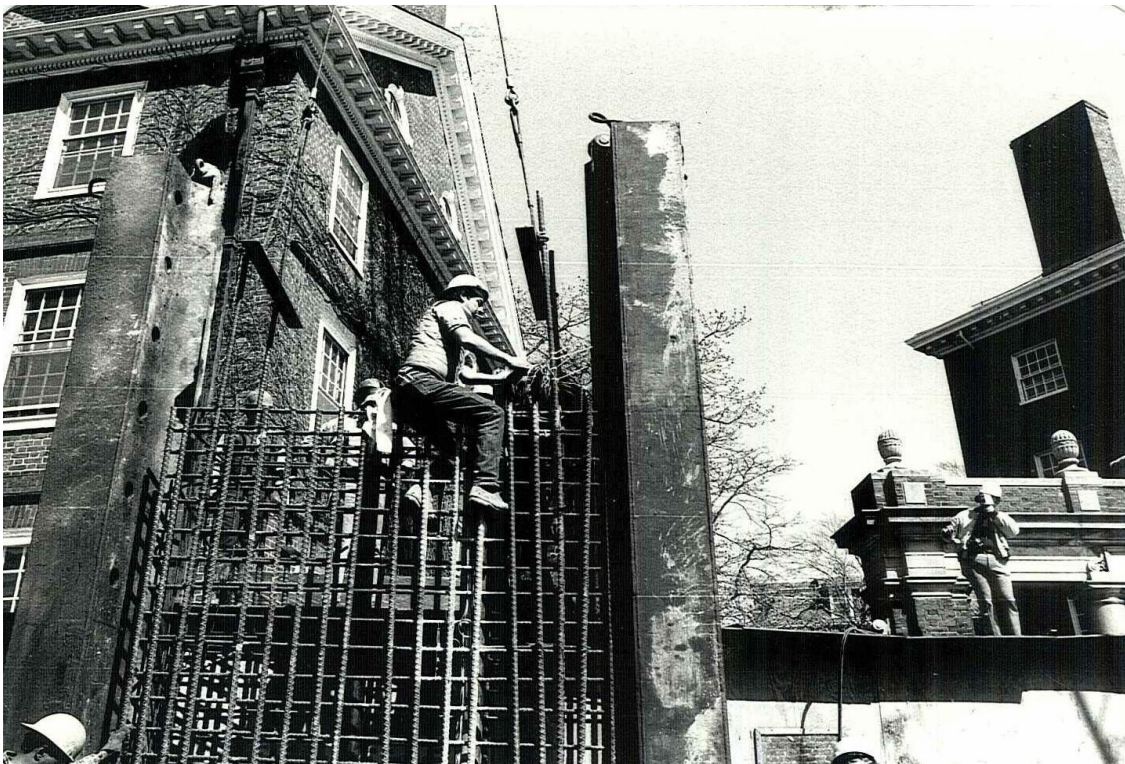
Photo 8: Temporary 'V' nose endstops.
