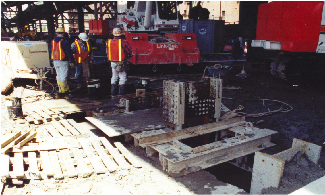
Photo 17: Soldier pile secured for splicing.
