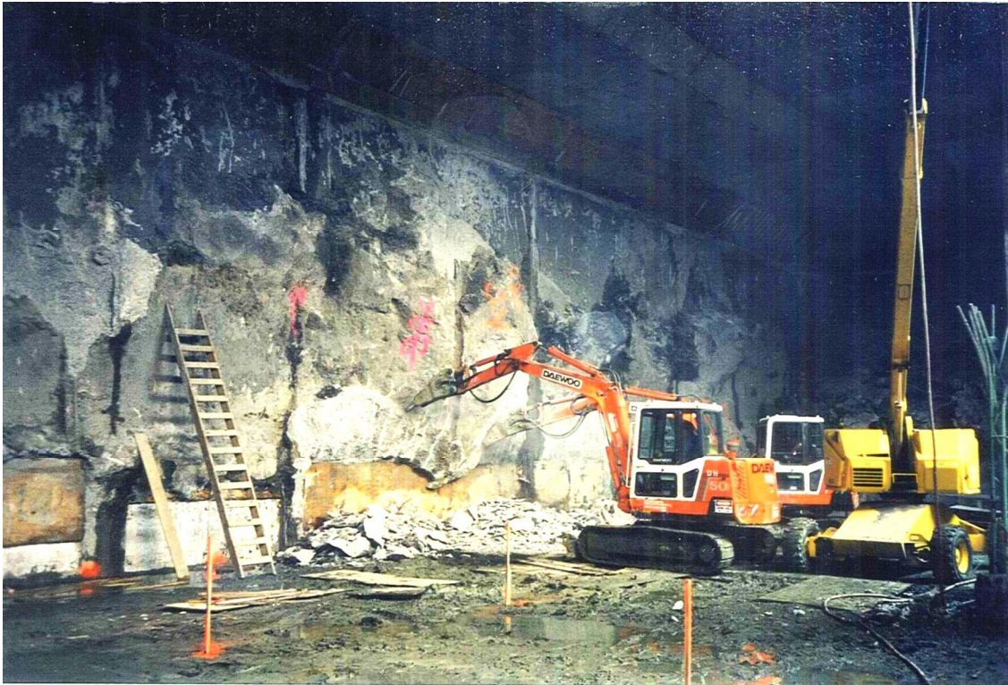
Photo 20: Chipping overpour concrete.
