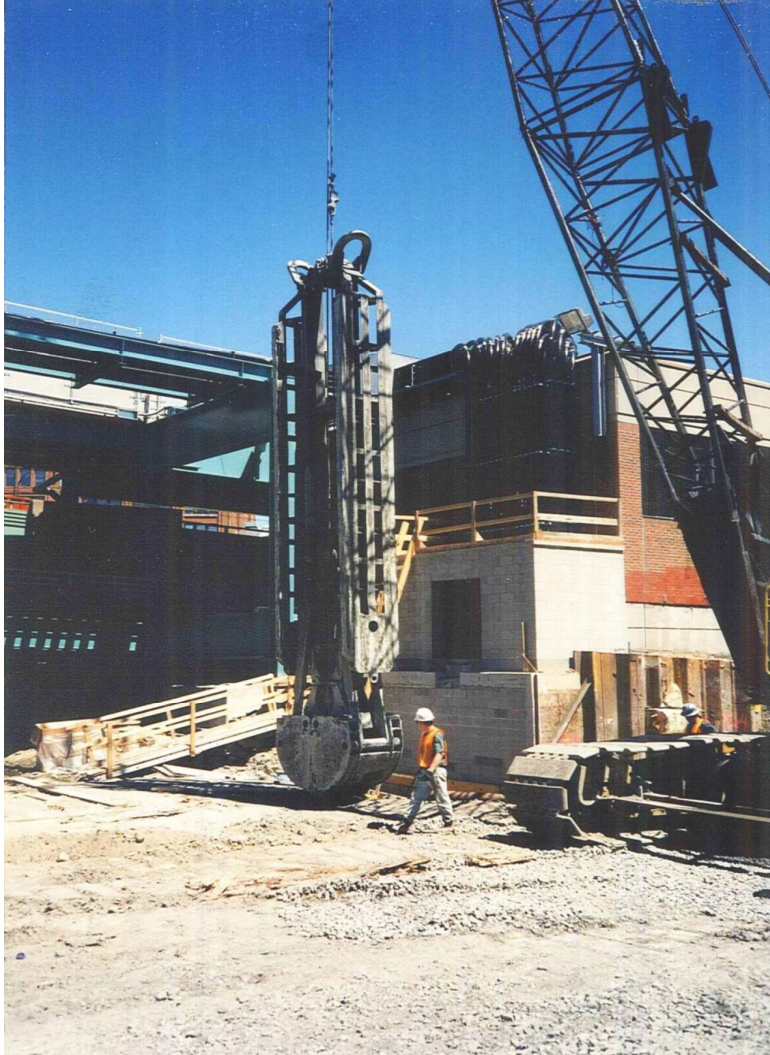
Photo 3: Typical cable suspended clam bucket.
