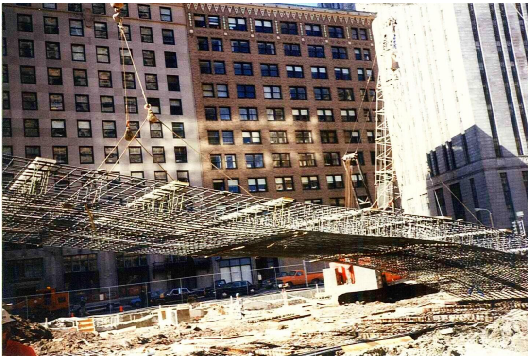
Photo 12: Hoisting cage, approx. 25' x 100' (note flexing at far right).
