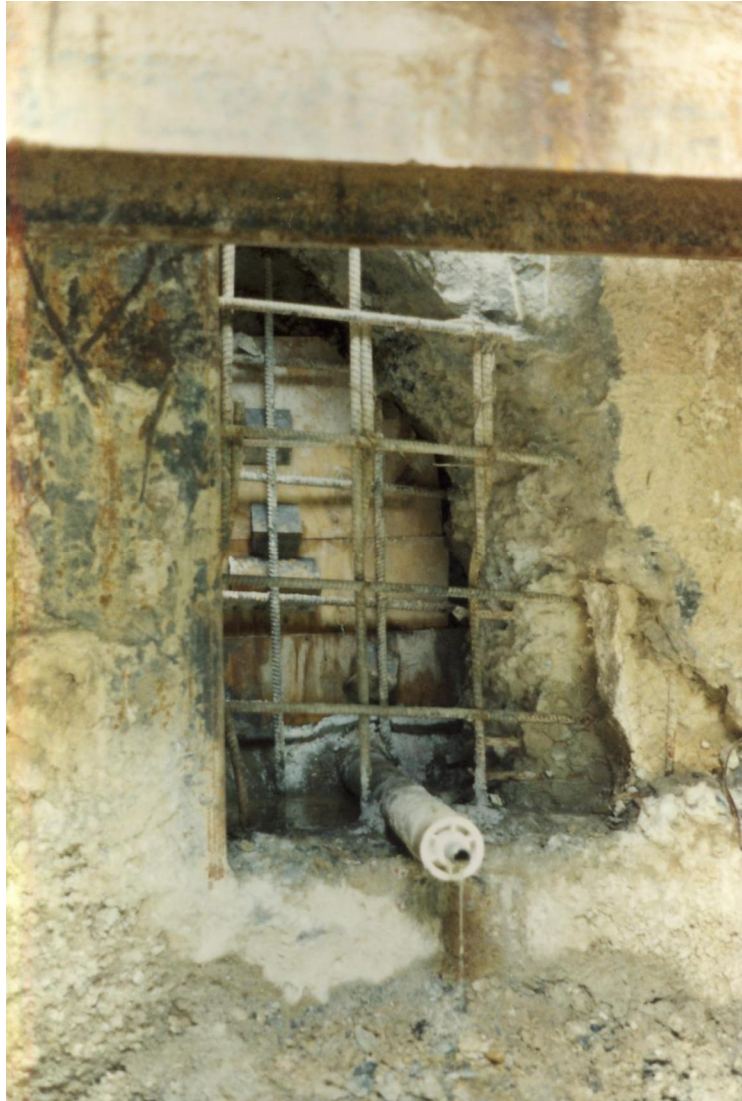
Photo 23: Repairing structural defect, debris removed, relieving water pressure to facilitate repair.
