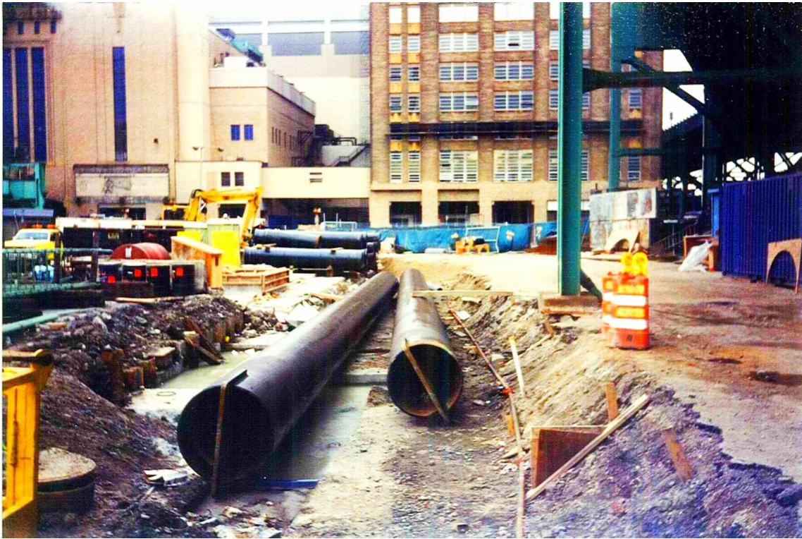
Photo 7: Temporary pipe endstops.
