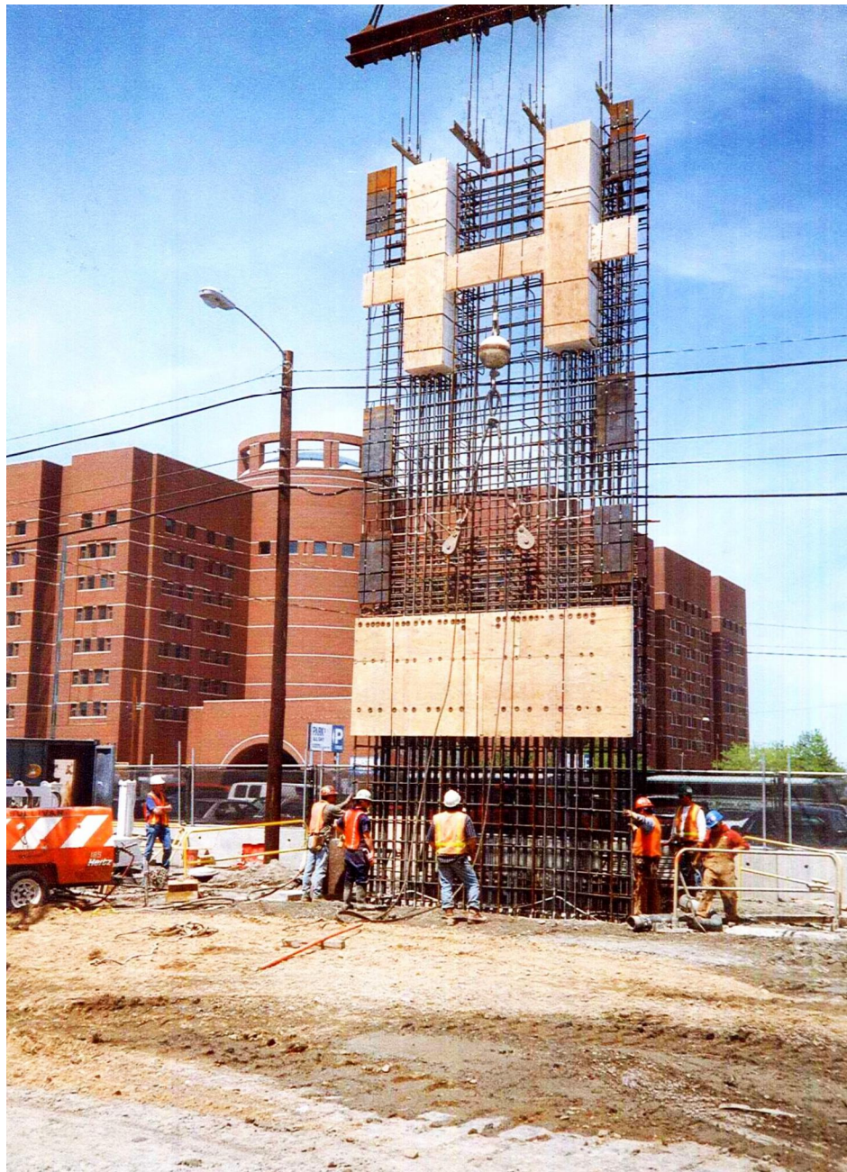
Photo 14: Lowering cage (note angles attached to vertical steel at top of cage, angles set on guidewall to support cage at design elevation).
