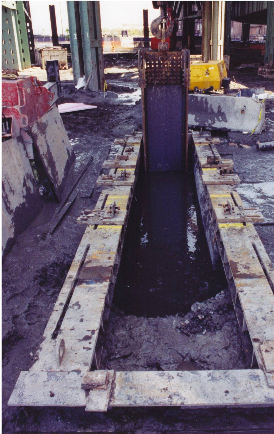
Photo 16: Soldier pile template to secure soldier piles.
