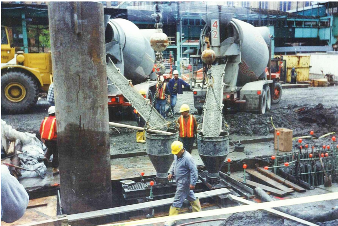
Photo 18: Concrete placement, sequential panel (one end-stop).
